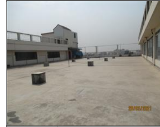
External photo(s) of the production unit(s) Rooftop.JPG
