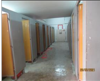
Photo of the sanitary facilities Toilet.JPG
