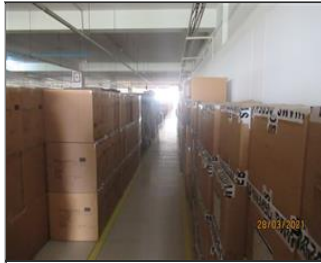
Photo of the inside of the main production hall Finished goods store.JPG
