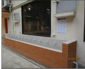
External photo(s) of the production unit(s) External hand washing point for COVID-19.JPG
